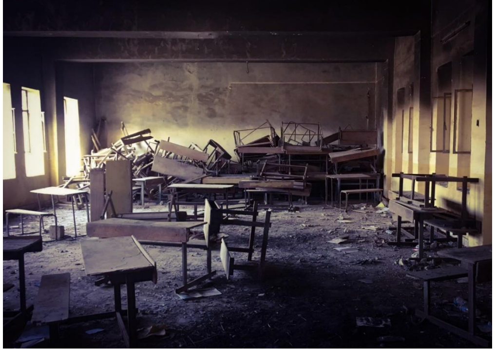
Destroyed school in Sulaiman Baig sub-district, Salah Al-Din Governorate. [Credit: OCHA Kirkuk Sub-Office]
