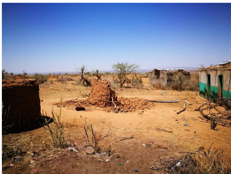
Figure 2 houses that were damaged during the violence. Photo Credit: OCHA/Ethiopia
