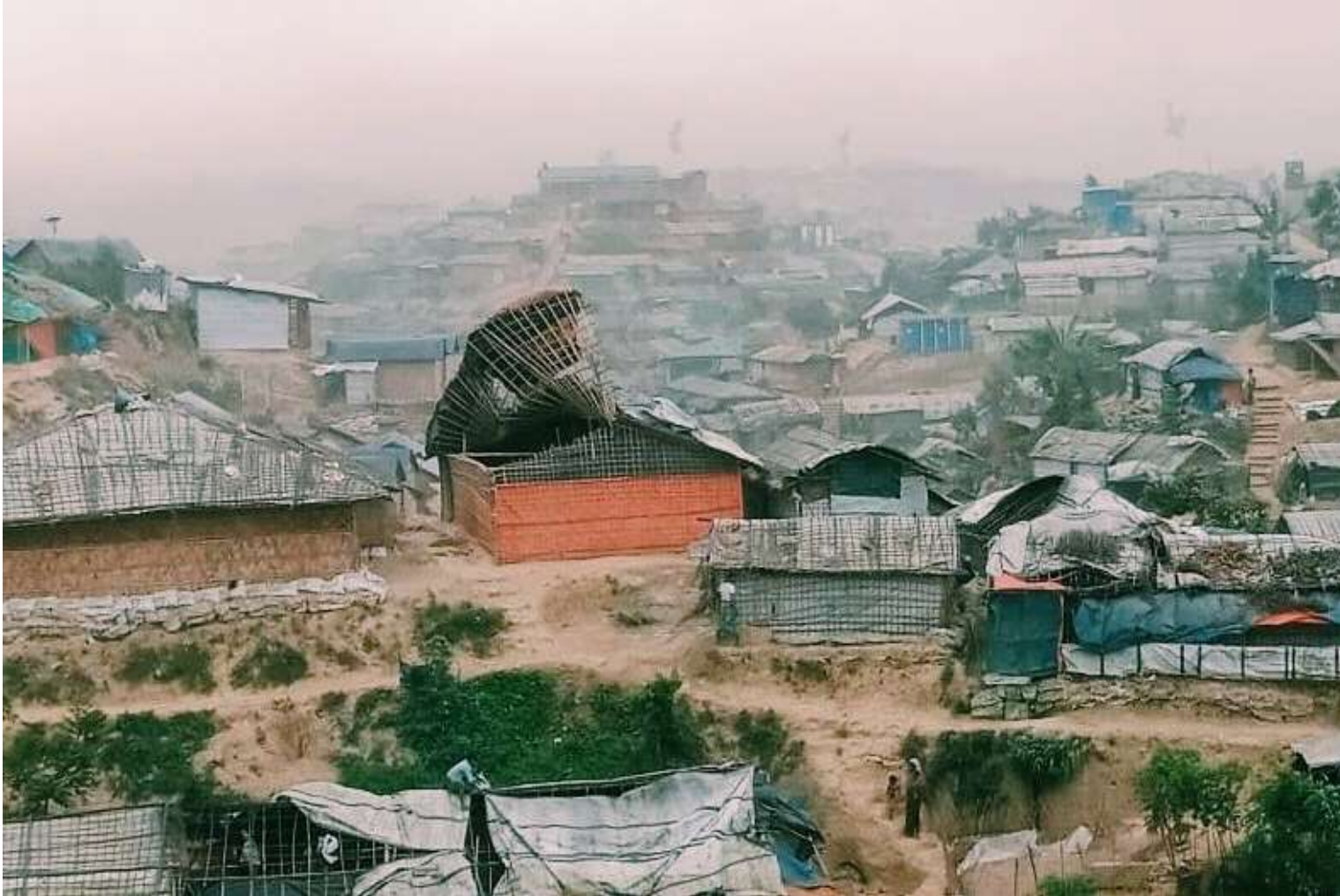
After Nor'Wester storm 25 th February, camp 18. (Photo credit: IOM)
