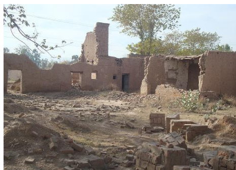
Credit: UNOPS Housing damage in Bara.
