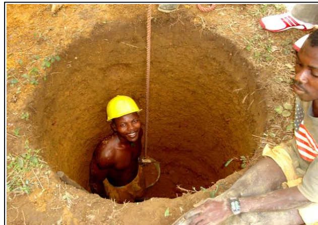
Photo 4: Well digging. / Courtesy: Norwegian Refugee Council
