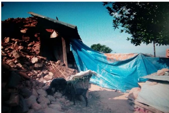
*Tarp insecurely attached to structurally unstable building in Devitar. Core messaging around safe tarp use and construction is necessary as distributions occur. SC staff are technically trained on this and will share this with beneficiaries of shelter kits and materials.*
